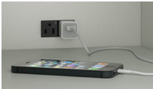
Interior Power Outlet
